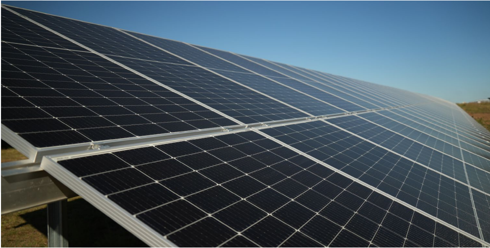
South Deep solar plant
