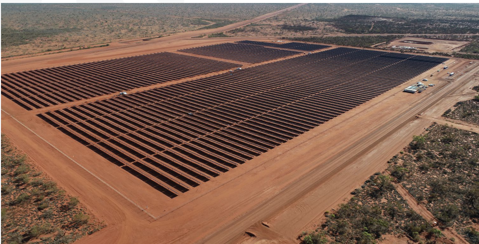
Gruyere solar plant
