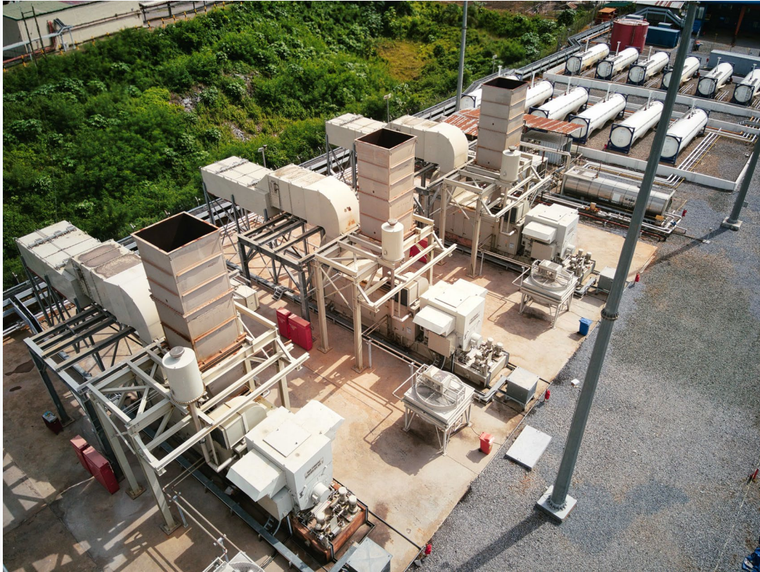
Genser gas plant at Tarkwa
