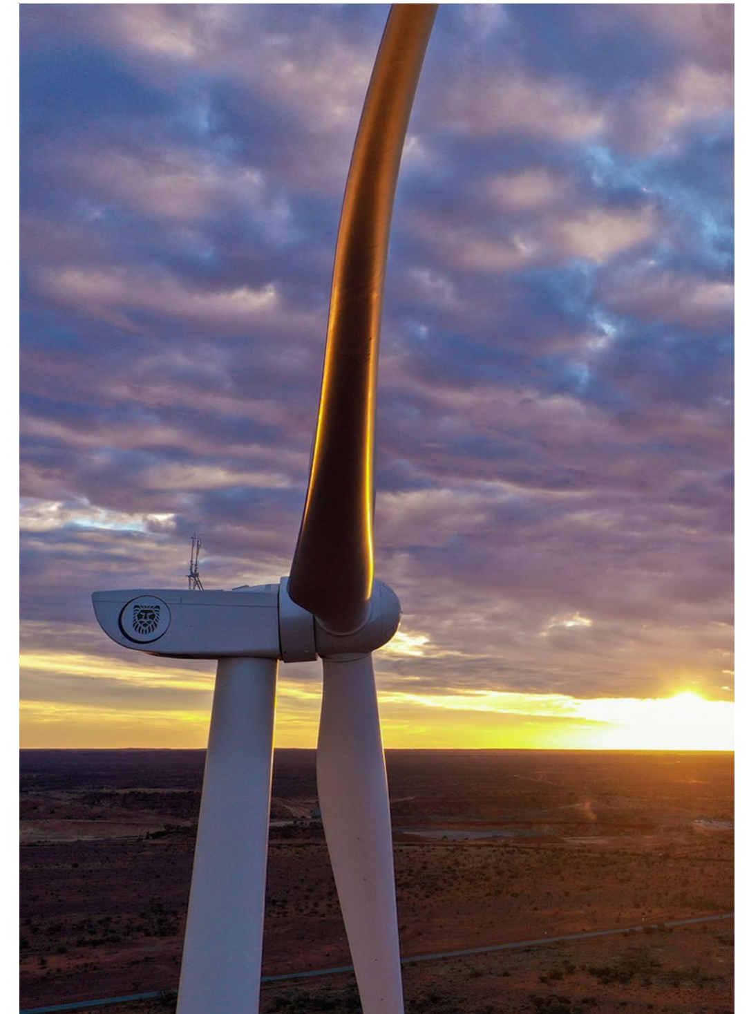
One of the five wind turbines at our Agnew mine in Western Australia
